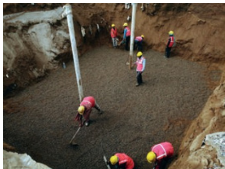
Step 2: Preparation of Base for Laying of High Quality Geotextile Sheets
