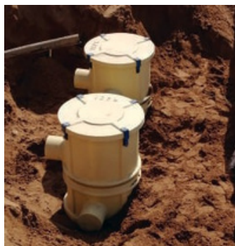
Step 6: Installation of Efficient Filtration Mechanism
