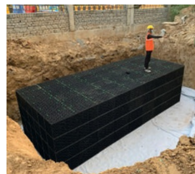
Step 4: Stacking of Polymer Modules for Installation of Rainwater Harvesting Tank
