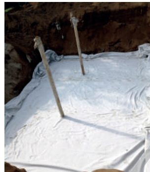
Step 3: Laying of Geotextile Sheets for Stacking of Polymer Modules
