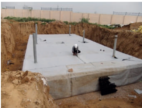
Step 5: Sealing of Geotextile Sheets after Installation of Polymer Modules
