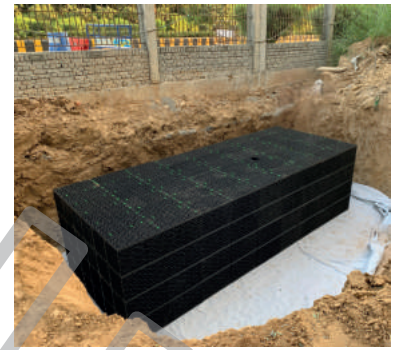
Step 4: Stacking of Polymer Modules for Installation of Rainwater Harvesting Tank
