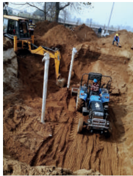
Step 1: Excavation is under process after Completion of Borewell
