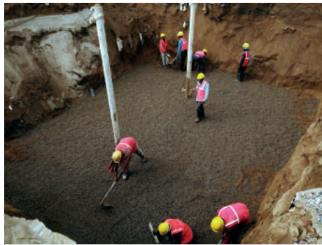
Step 2: Preparation of Base for Laying of High Quality Geotextile Sheets
